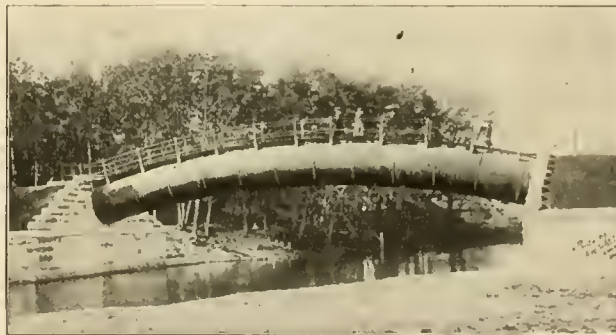
A PIPE BRIDGE.
